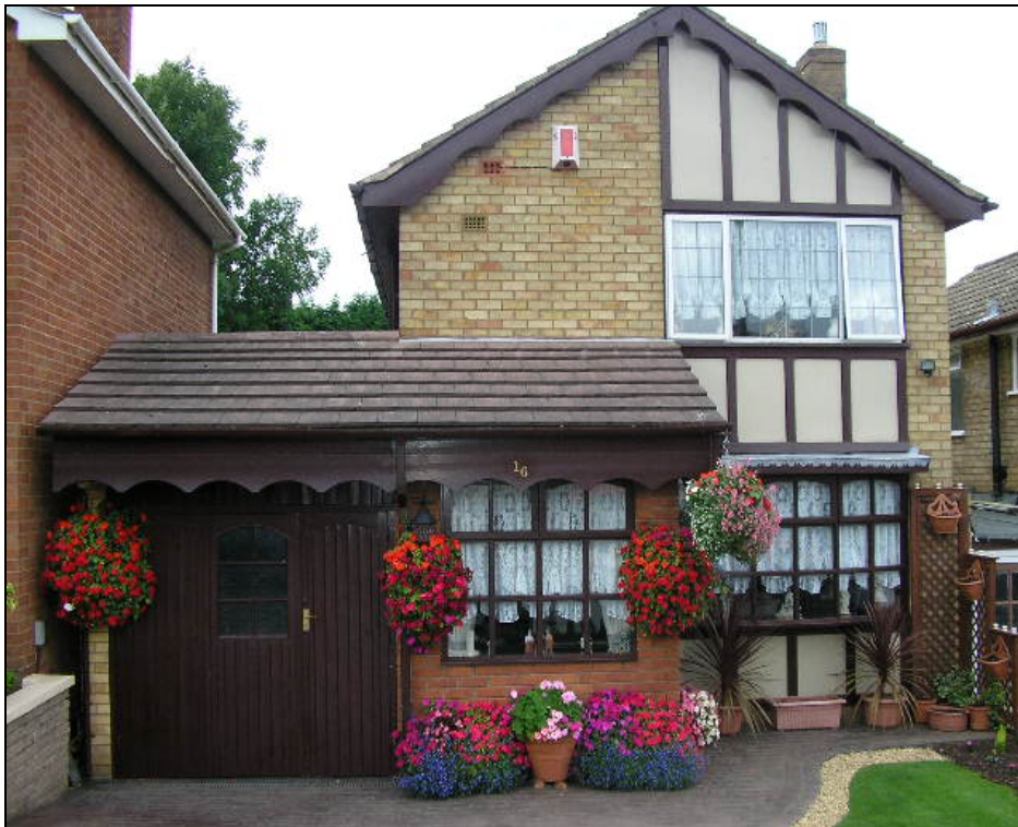
View showing the front elevation adjoining property No. 17 Westminster Road to the west of the application property
